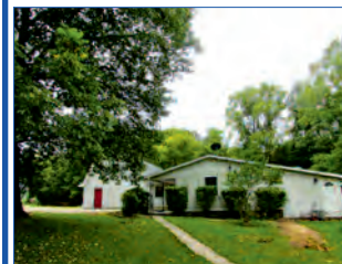
511 W QUARRY ROAD, ORLEANS
